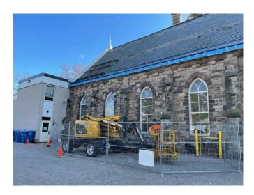
You can see the phases, as they remove the old roof, insert the new ends of the trusses and then install the new roof (blue) and fascia.
